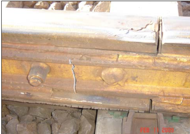
Figure 4. IJ Failed Due to Cracked Bar at 1,090 MGT
