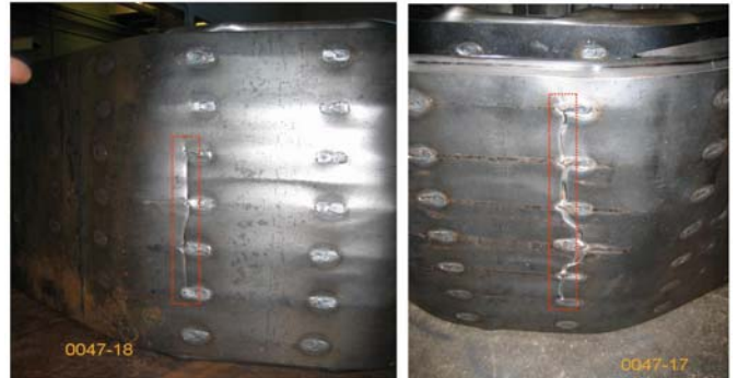
Figure 21. Cracks in Inner Facesheet of 0047-18 (left) and 0047-17 (right)
