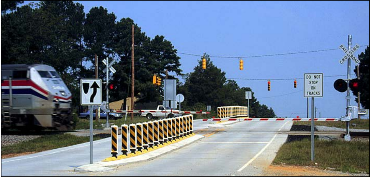
Figure 1. Traffic Channelization Device Installation at Highway-Rail Grade Crossing (photo courtesy of NCDOT)
