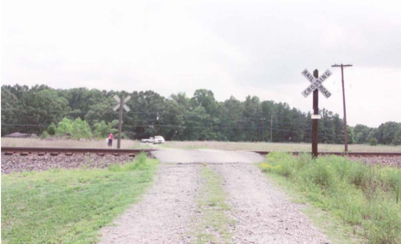
Figure 5. Private Grade Crossing Cross Buck Sign Treatment (16)
