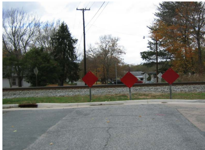
Figure 3. View of a Sample Crossing Closure Treatment (Volpe Center)
