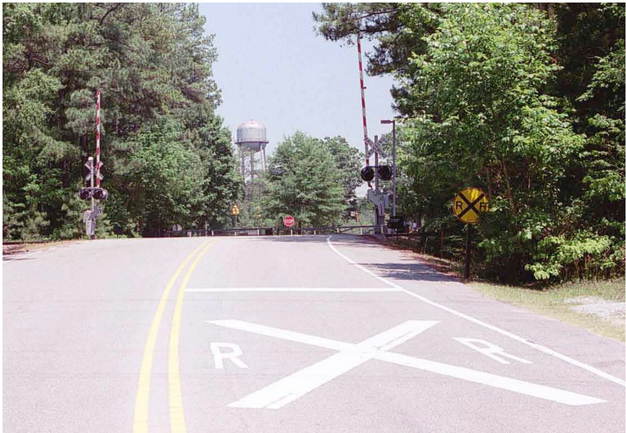
Figure 7. Private Grade Crossing Gate, Flashing Light, and Pavement Markings Treatment (16)
