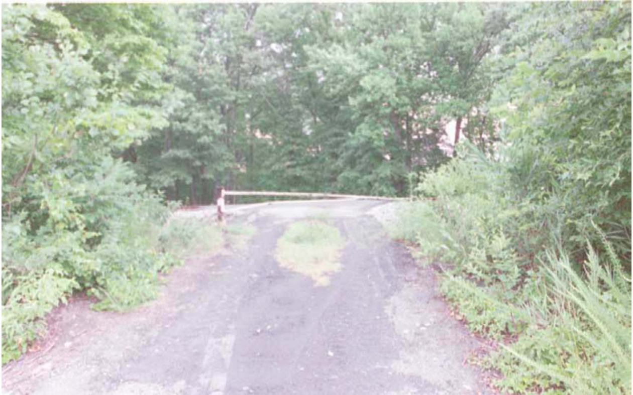
Figure 6. Private Grade Crossing Gate with Locking Mechanism Treatment (15)
