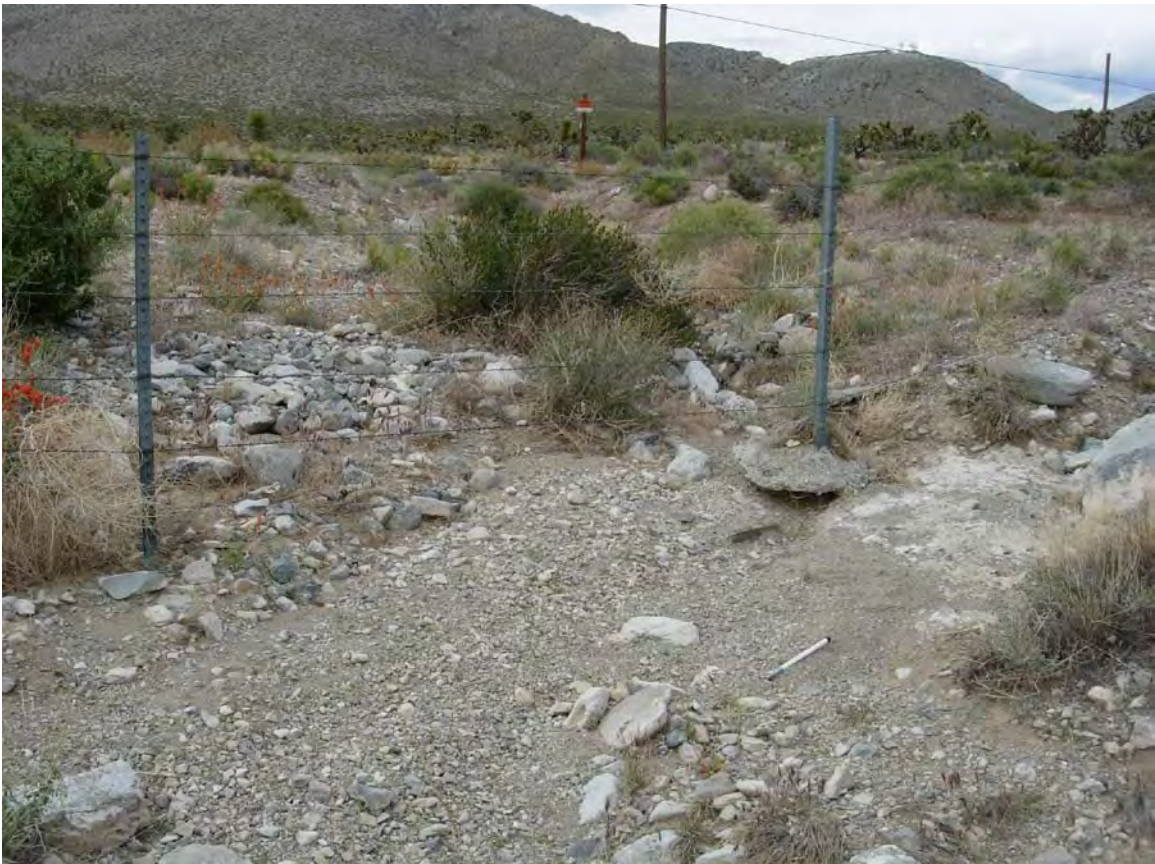
Exhibit A. Figure 18. Manmade drainage connecting to road culvert within HUC 8 Death Valley Lower Amargosa / HUC 12 Piute Valley Subwatershed
