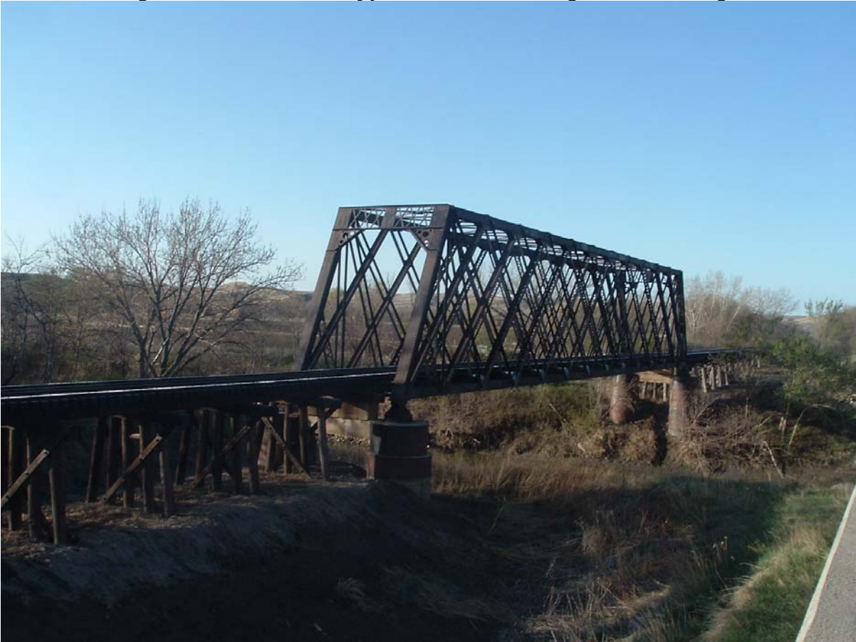
Figure 7-2. Photo of Typical DM&E Through-Truss Bridge
