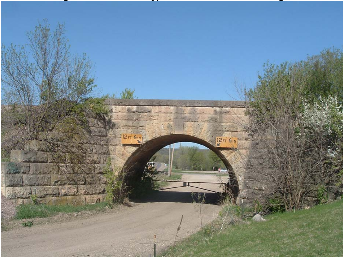
Figure 7-3. Photo of Typical DM&E Stone Arch Bridge
