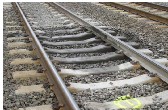
Figure 5. Mud Spot That Caused High Acceleration Levels
