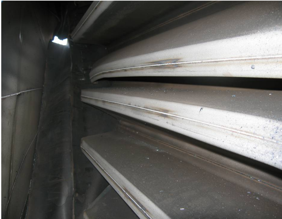
Figure 275. Separation of the outer face sheet on the end EMS structure.
