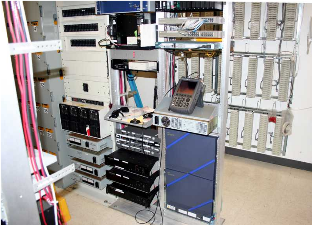
Figure 46: BNSF Auburn BS rear view of three base station radios, bottom center
