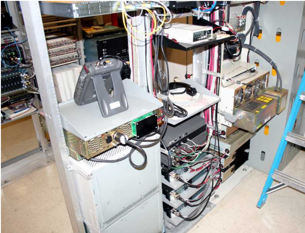
Figure 46: BNSF Auburn BS rear view of three base station radios, bottom center
