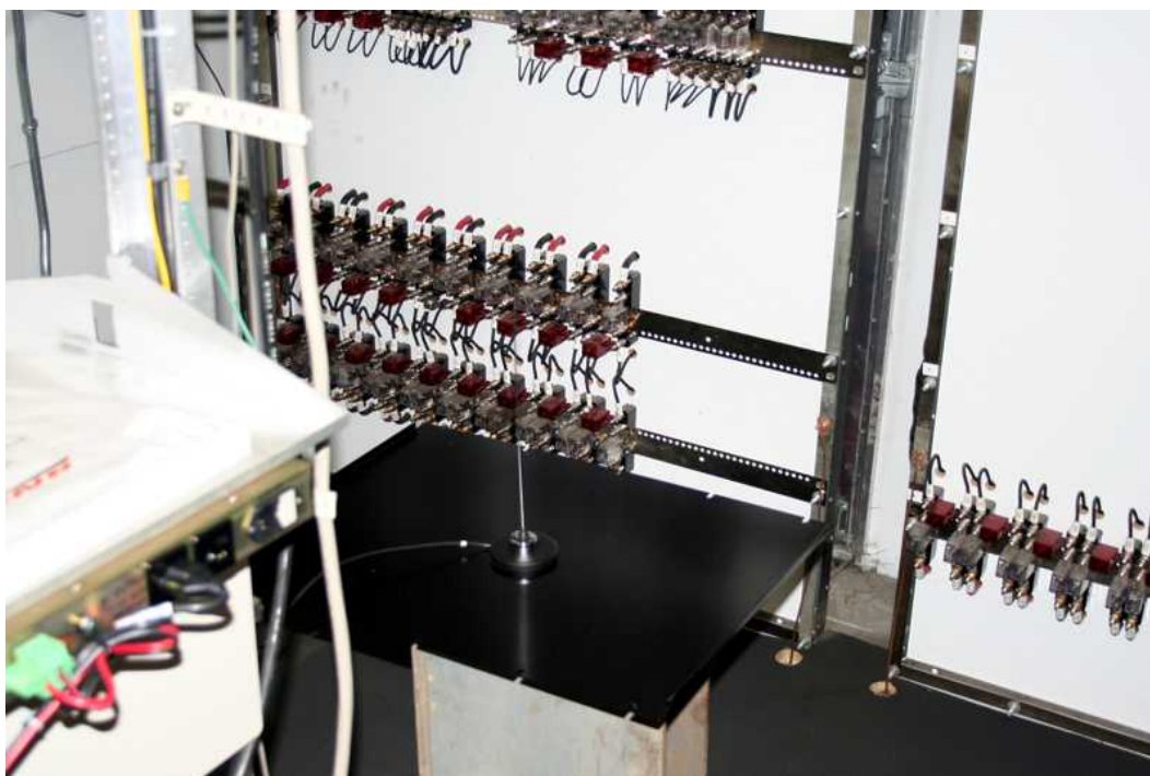
Figure 10: BNSF CP Boeing interior view with 220 MHz antenna and metal ground plane
