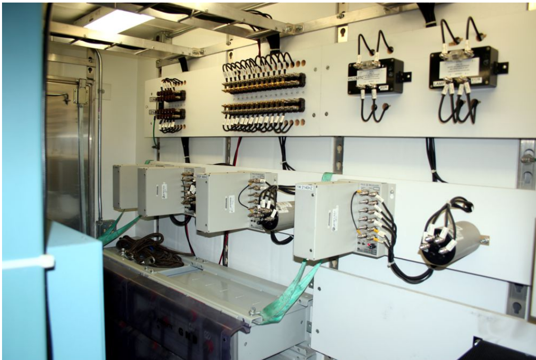
Figure 29: BNSF CP Titlow interior view with audio frequency track circuit equipment
