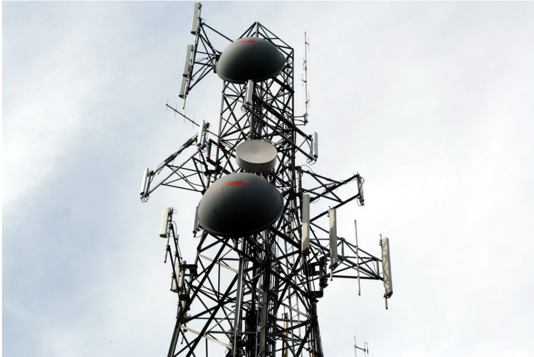
Figure 43: BNSF Auburn Base Station antennas mounted on side of tower
