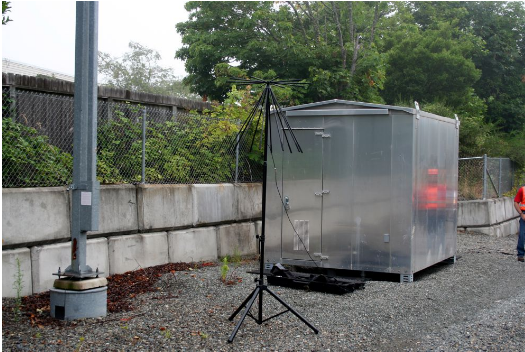
Figure 27: BNSF CP Titlow view of 35' swing-down antenna mast for 160 MHz ARES radio
