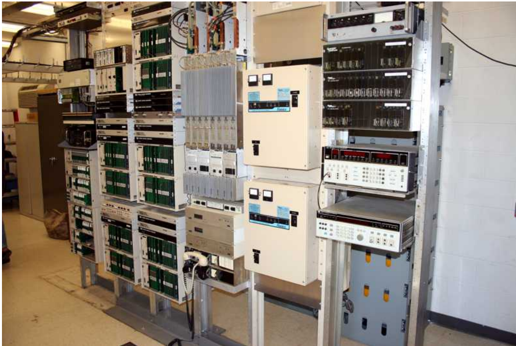
Figure 47: BNSF Auburn Base Station microwave equipment
