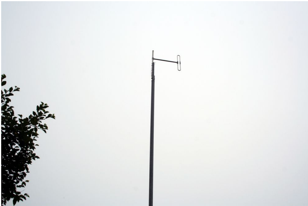
Figure 27: BNSF CP Titlow view of 35' swing-down antenna mast for 160 MHz ARES radio
