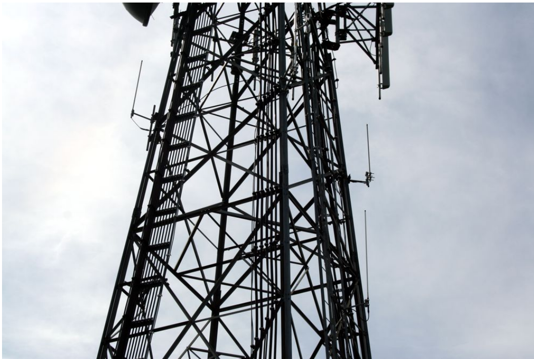
Figure 43: BNSF Auburn Base Station antennas mounted on side of tower
