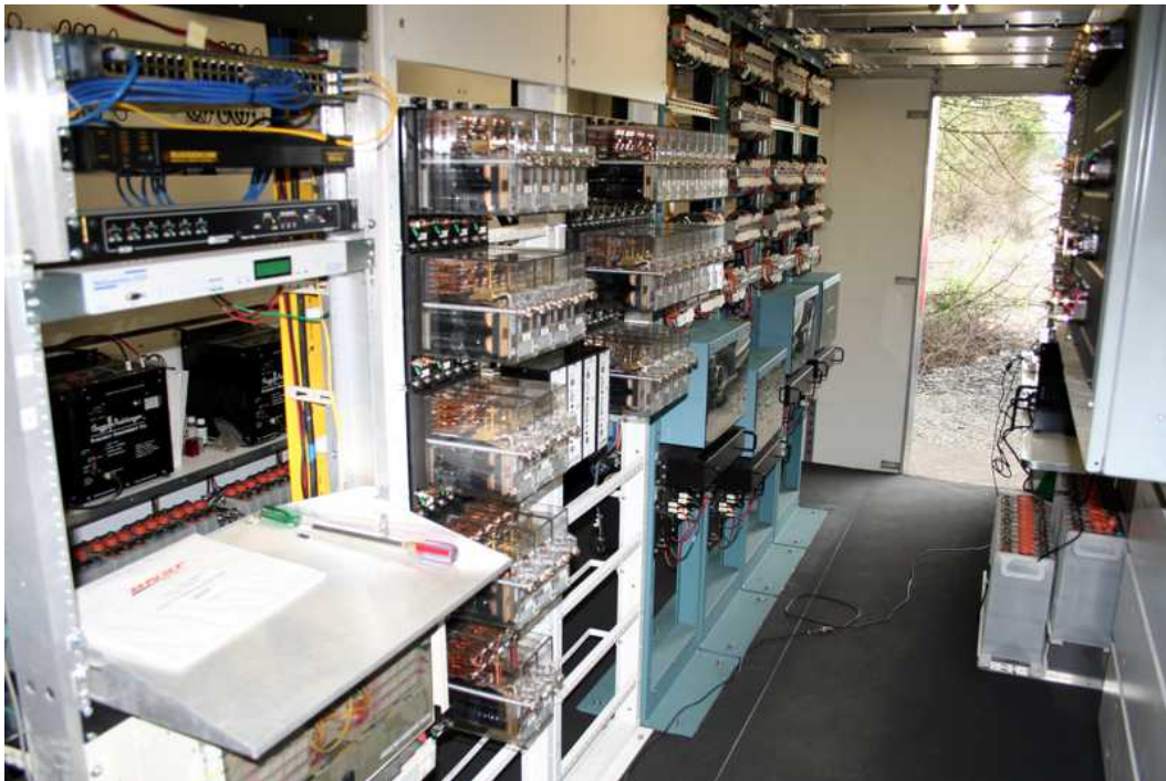
Figure 8: BNSF CP Boeing interior view with DC track circuit relays
