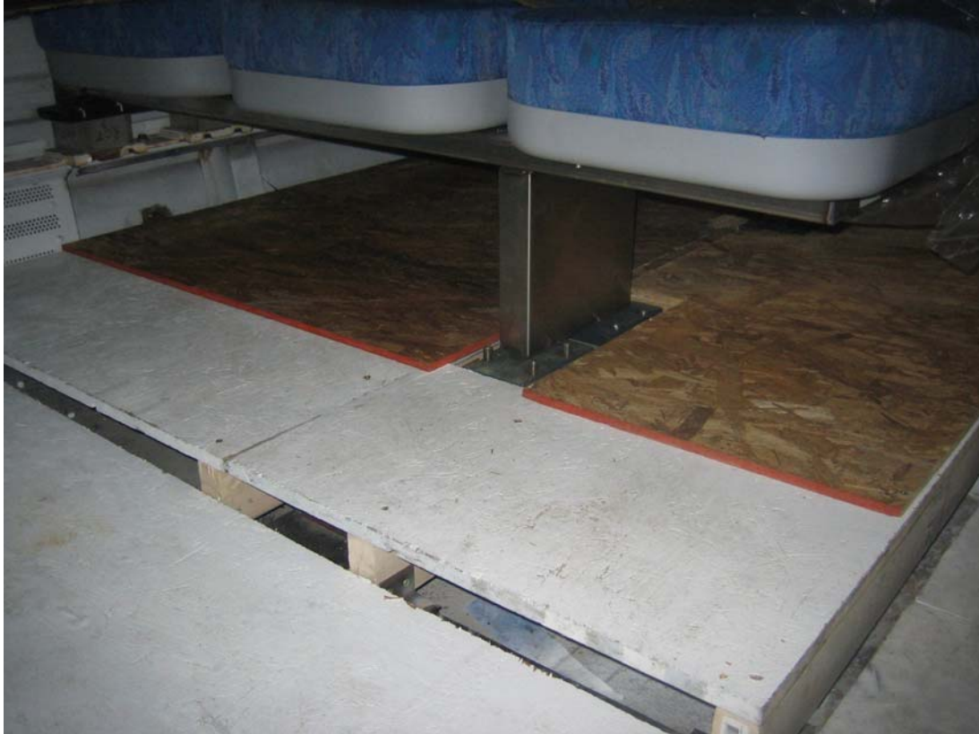
Figure 8. Plywood Floor Installed around the Seat Installation Raising the Floor to the Level Where the Pedestal Base is Installed in Experiment 1.1
