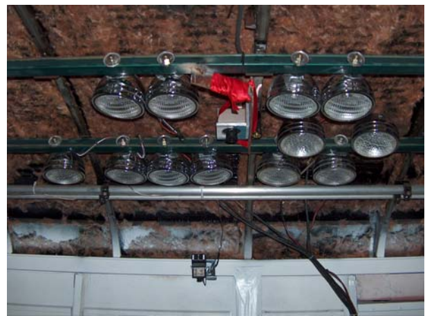
Figure 41. One U512 Camera and 24 Flood Lights Were Installed along the Wall and One U512 Camera and 12 Lights Were Installed along the Ceiling
