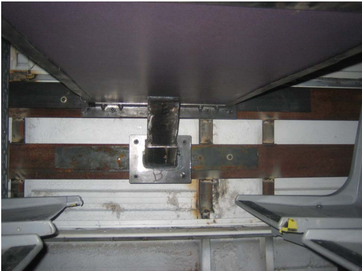
Figure 17. Two 20-Foot Bars were Welded Four Inches Apart on Top of Vertical Bars
