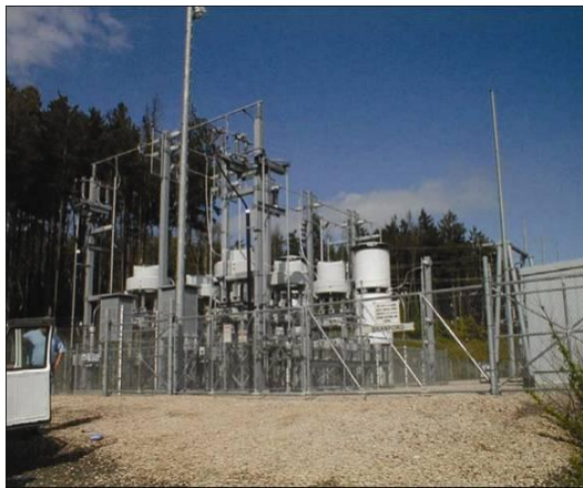
Figure 2-14 Traction power substation
