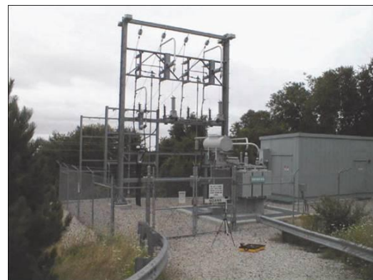
Figure 2-16 Paralleling station
