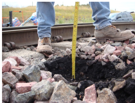
(b) Coal dust just beneath top of ballast
