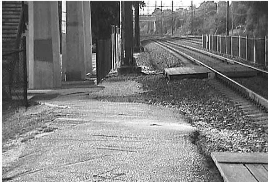
Figure 5-3. Photograph of Halethorpe Station, Halethorpe, MD, Showing Narrow (6 feet wide) Southbound Platform Adjacent to High-Speed Track No. 3
