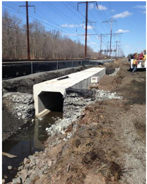
Track and Structure Upgrades
