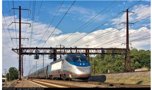
Traction Power Upgrades
