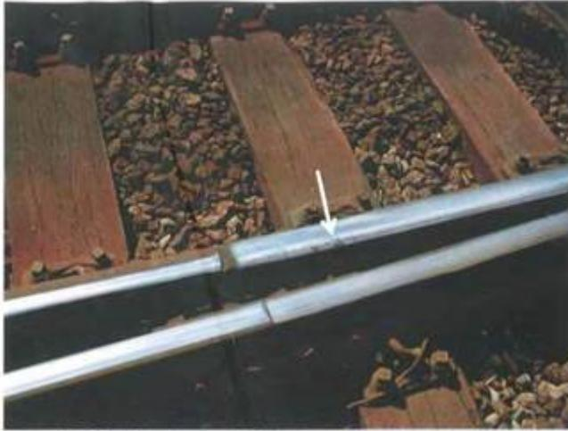
Figure 1. GCC and contact band shift due to canted and uncanted rail and joint misalignment.
