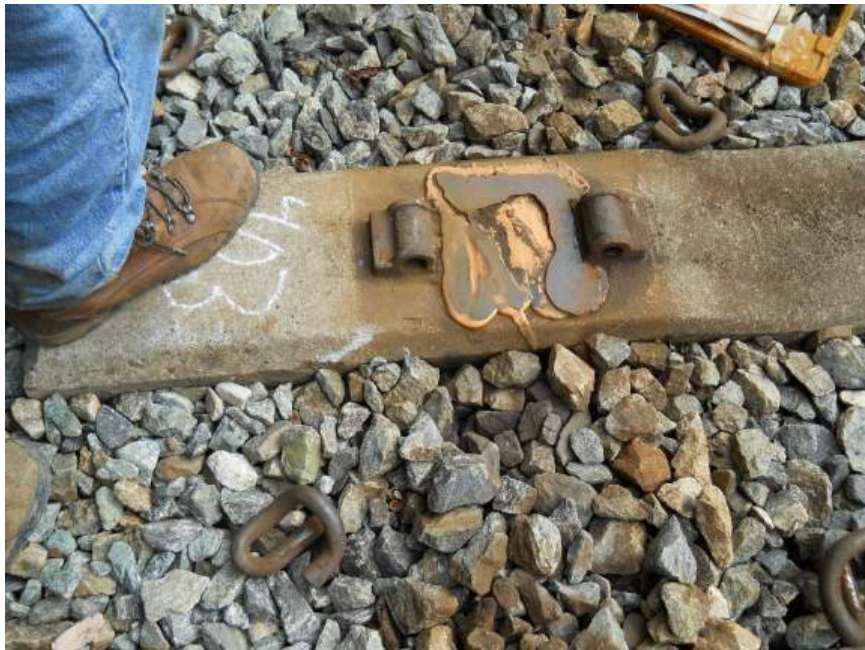
Figure 24. Curve 17, View of Rail Seat Previously Repaired
