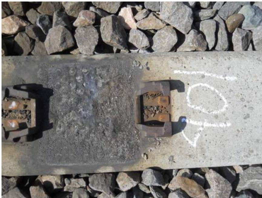
Figure 43. High Rail Seat of Tie 401 on Curve at MP 12.8
