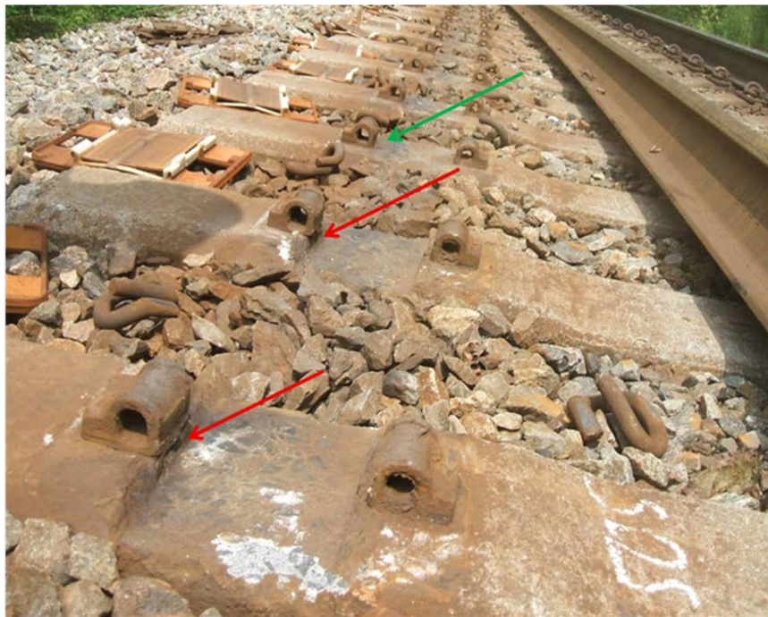
Figure 4. Example of Ties Shown in Figures 2 and 3 with Rail Removed, Showing Depth of RSA
