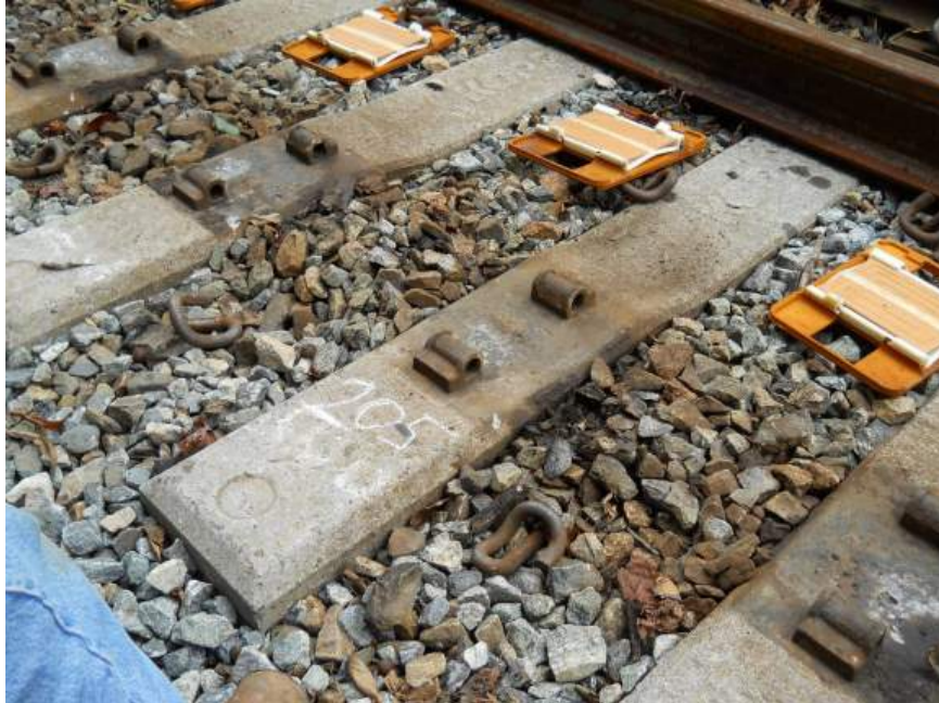
Figure 23. Curve 17, Typical Rail Seat Conditions near Tie 205
