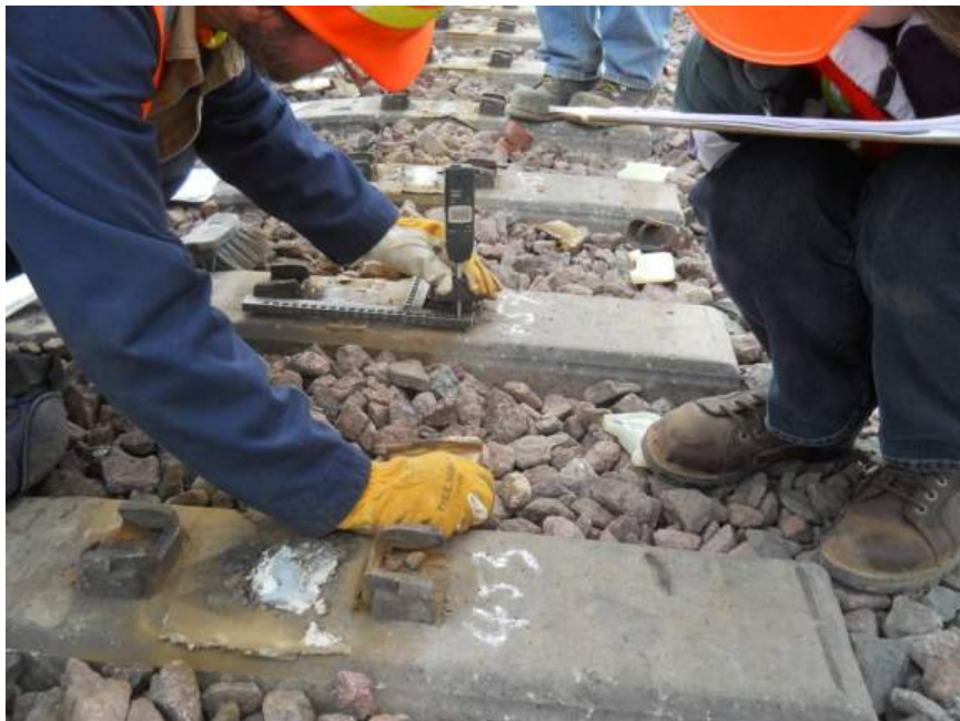
Figure 9. After Old Pads Have Been Removed, the Rail Seats Are Exposed
