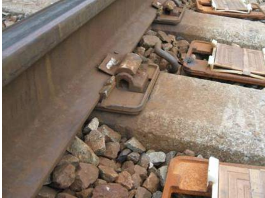
Figure 3. Another View of the Same General Location as Shown in Figure 2; Ties Reported to Have RSA, but with Rail in Place It is not Feasible to Measure RSA Depth
