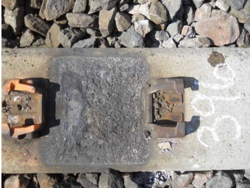
Figure 42. High Rail Seat of Tie 396 on Curve at MP 12.8
