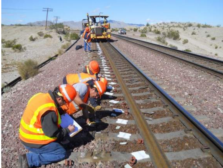
Figure 10. View from Figure 9 Looking Back to the Machine Repairing Rail Seats and Placing Pads in Position
