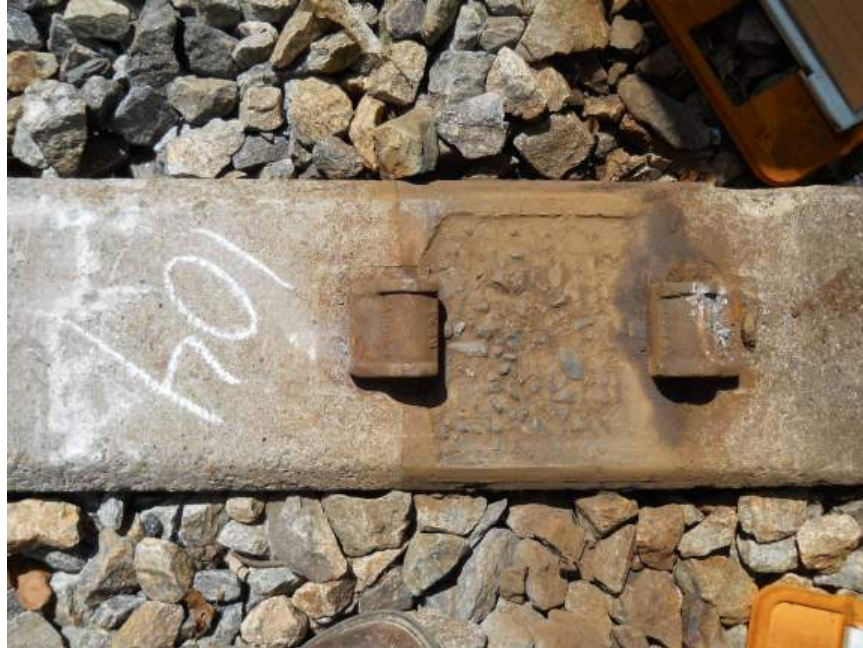
Figure 25. Curve 16, Tie 104, Left Is Field Side, with More RSA Depth on the Field Side of the Rail Seat, and It Results in Outward Tilt (cant) of the Rail
