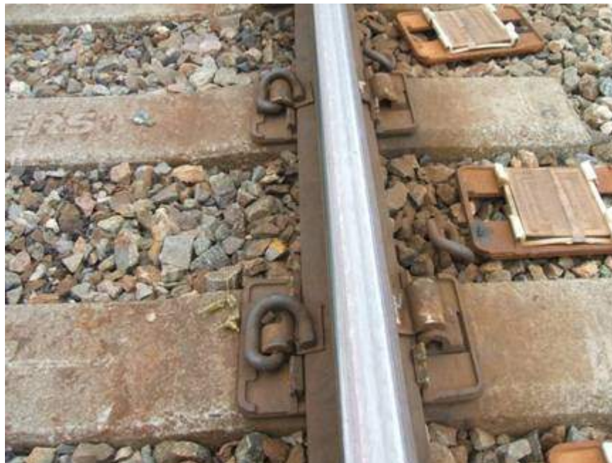
Figure 2. Example of Ties Reported to Have RSA, but with Rail in Place It is not Feasible to Measure RSA Depth
