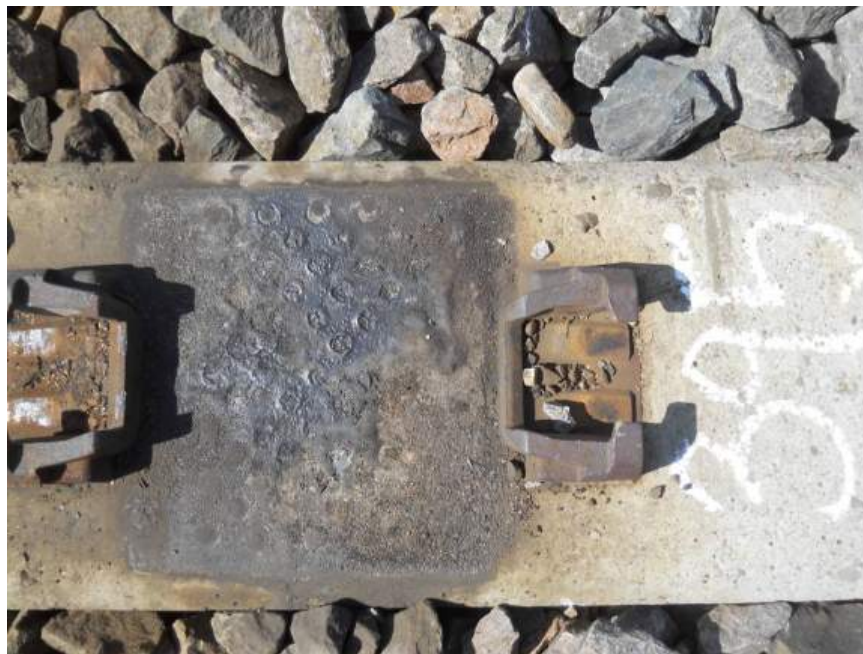
Figure 41. High Rail Seat of Tie 395 on Curve at MP 12.8
