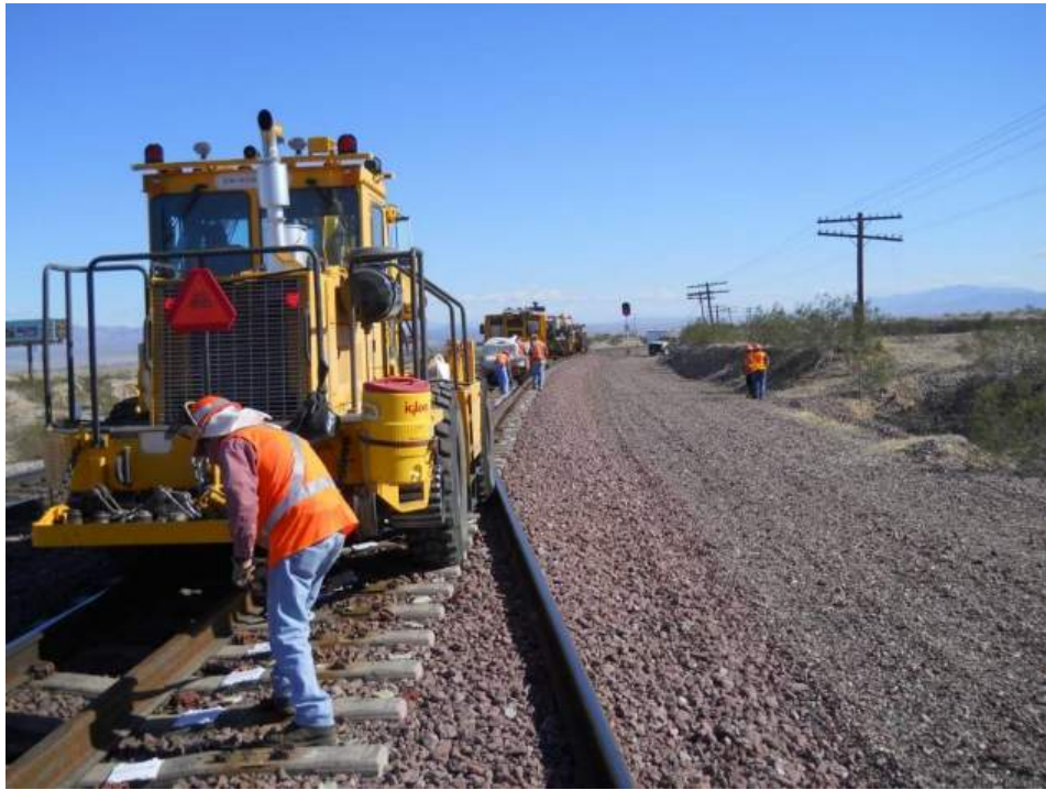
Figure 7. Typical Maintenance Gang Conducting a Rail Change and RSA Repair (Existing, old rail is being removed and set to the field (outside, right) side of track. Note new rail has already been placed in the center of the track.)
