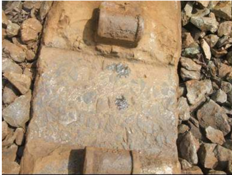
Figure 1. Example of Severe RSA
