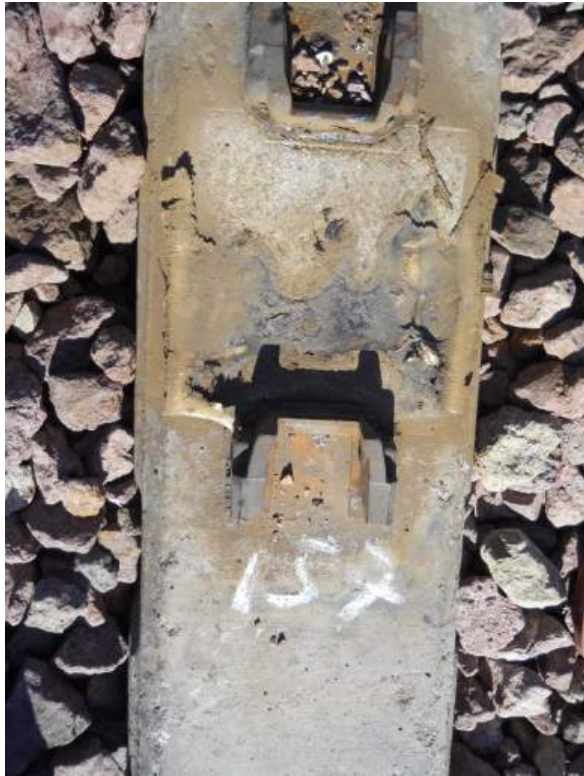
Figure 31. MP 584.5 Typical RSA in Curve, Tie 126, and Tie 157 (Gauge side is at top of photo and shows gauge side with deeper abrasion than field side, confirming inward tilt (cant).)
