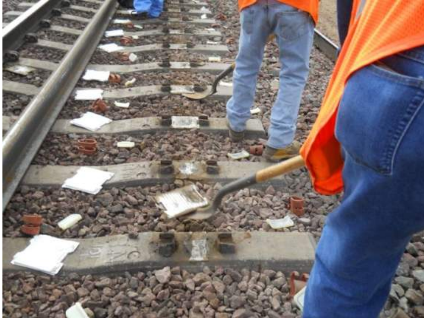
Figure 8. Following the Rail Removal (Figure 7), Old Pads Are Removed and the Rail Seat Is Scraped Clean
