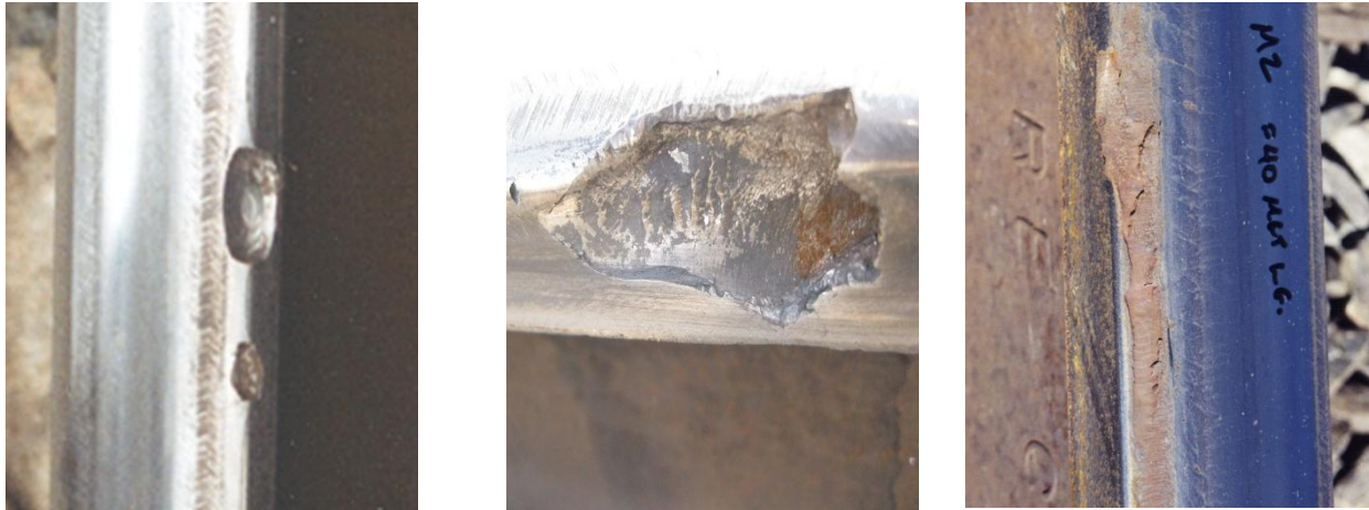
A) Loss of rail cant due to rail seat abrasion resulted in overloading of the gauge corner B) Well-lubricated rail with a sharp gauge corner C) Gauge corner collapse in a dry environment
