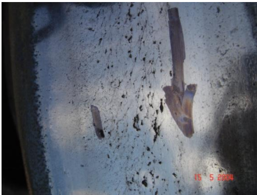
C) Well-defined cracks on the field/rim side of the wheel.
